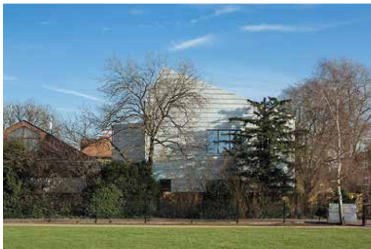
Figura 3.3 – New Studios, Wimbledon College of Arts - Perroyre & Prasad (fonte: https://www.penoyreprasad.com/project/new-studios-wimbledon-college-of-art/ )
