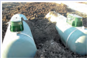
Serbatoi gas interrati
